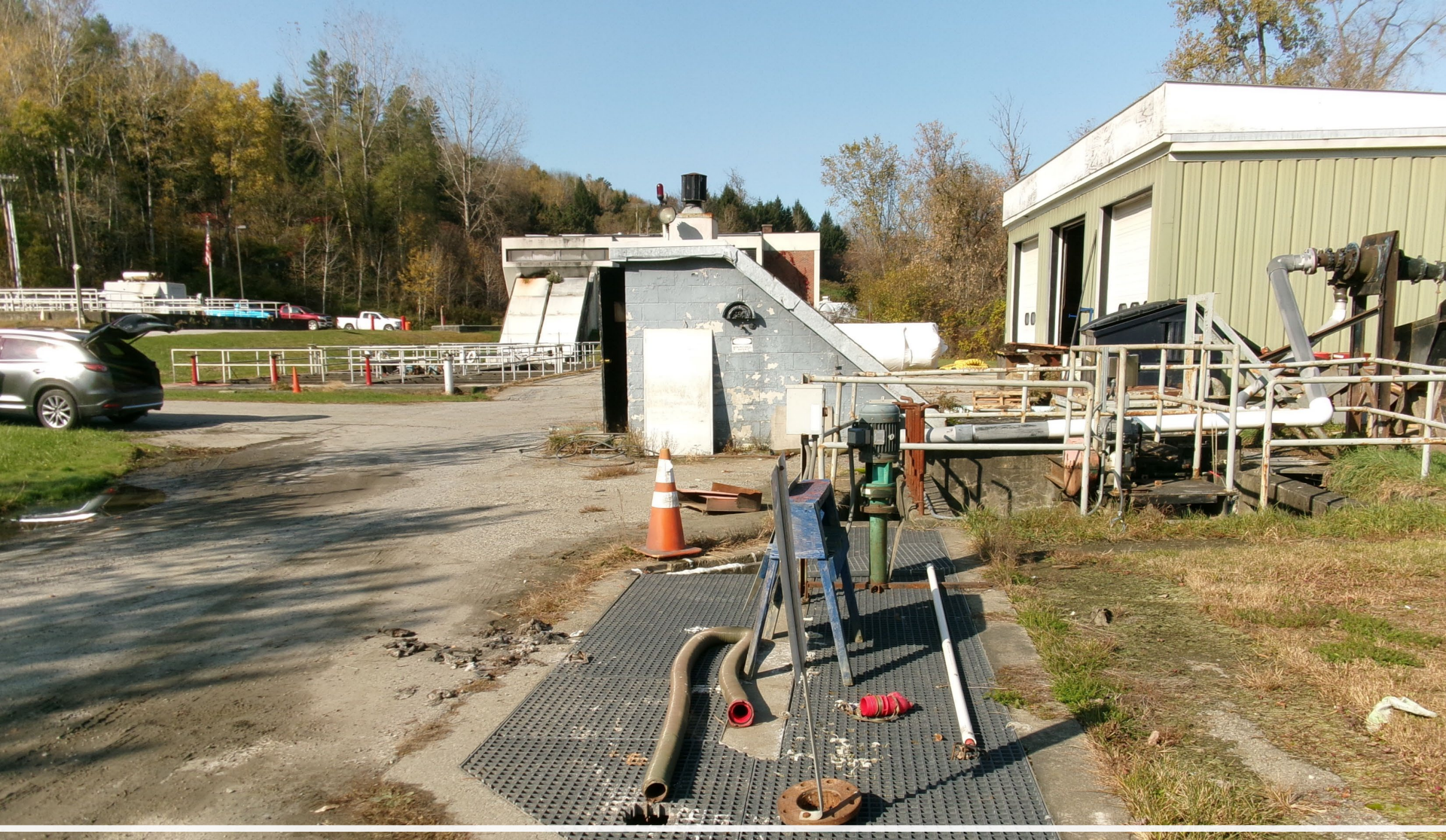
Existing Comminutor Structure
