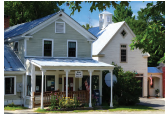
ADUs can accompany a variety of principal buildings, as here in the carriage house above a garage in Corinth, Image credit: Richard Amore
