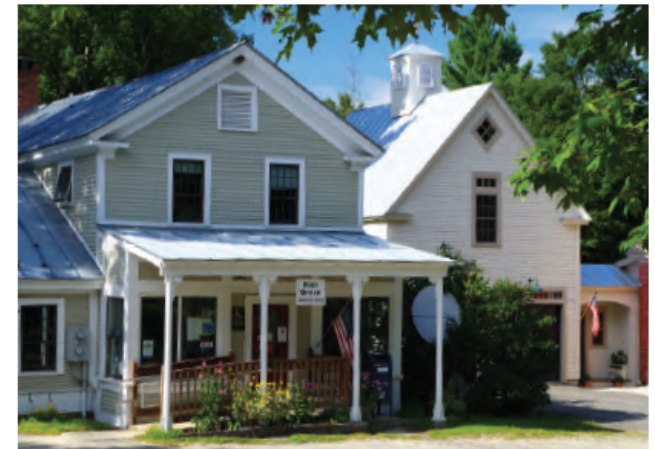
ADUs can accompany a variety of principal buildings, as here in the carriage house above a garage in Corinth, Image credit: Richard Amore
