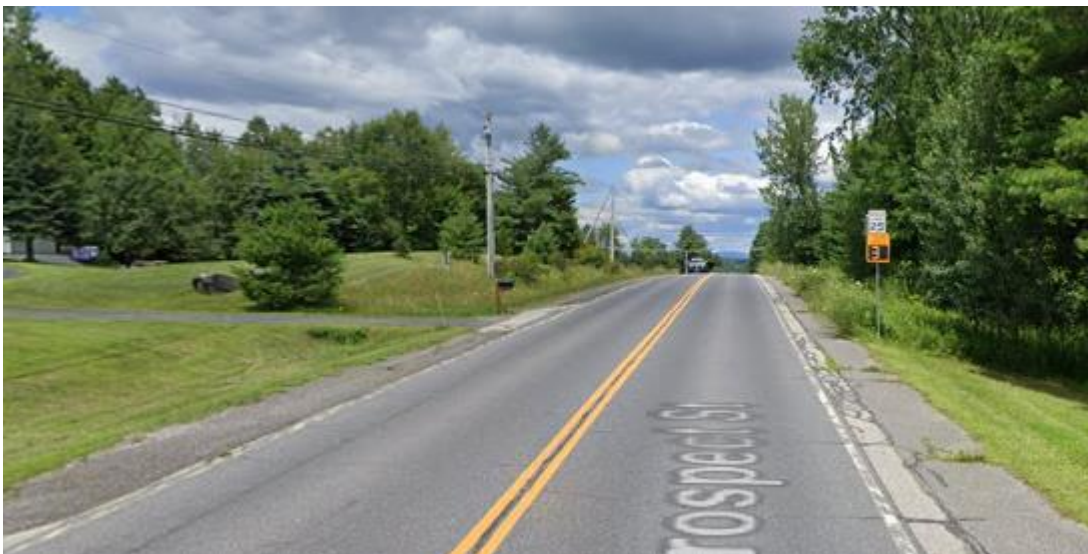
Figure 1 Google Maps image of Prospect Street south of City line – includes edge lines and radar speed feedback sign
